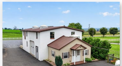
30x48 Warehouse & Office
