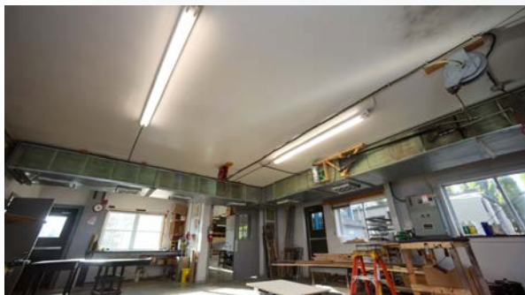
Banza Air Makeup System With Ductwork
