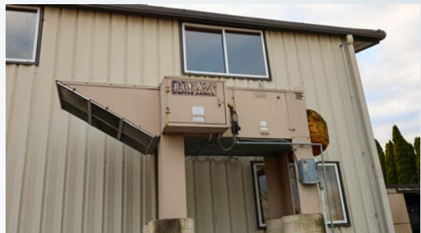
Banza Air Makeup System With Ductwork
